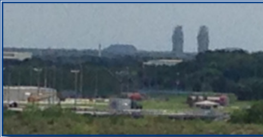
Launch pads, Cape Canaveral, Florida
